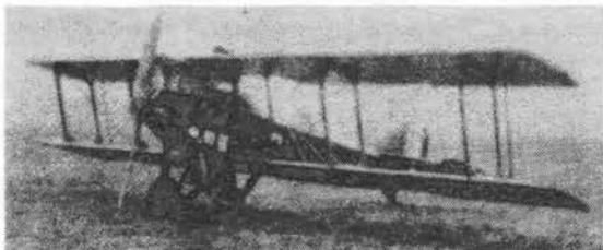
Le Pere with Supercharged Liberty Engine
