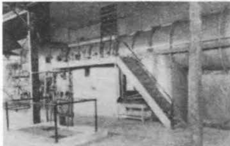
Section of Wind Tunnel, Showing One Control Board and Fan
