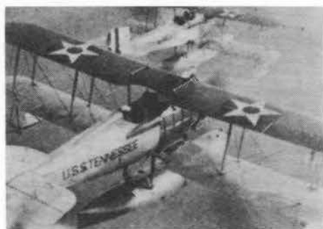
UO-1 and VE-7 Vought Shipboard Planes. Aircraft Catapults Shoot Them into Air with Such Velocity They do not Touch Water When Launched From Battleship's Deck
